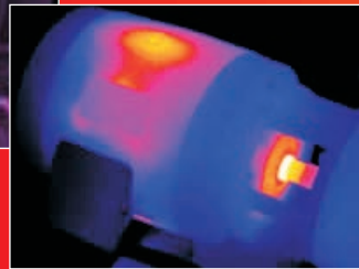
Incipient motor winding damage
